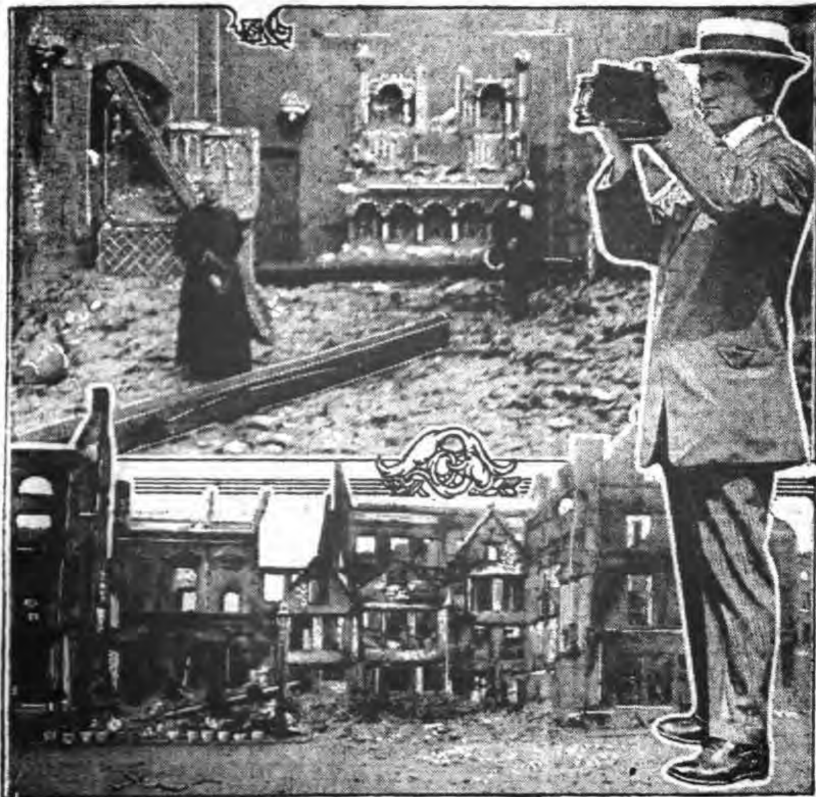
UPPER—INTERIOR OF WRECKED CHURCH IN TERMONDE; LOWER—ROW OF SHELL RIDDEN HOUSES IN TERMONDE; ON RIGHT—ADRIAN C. DUFF AND HIS CAMERA.
